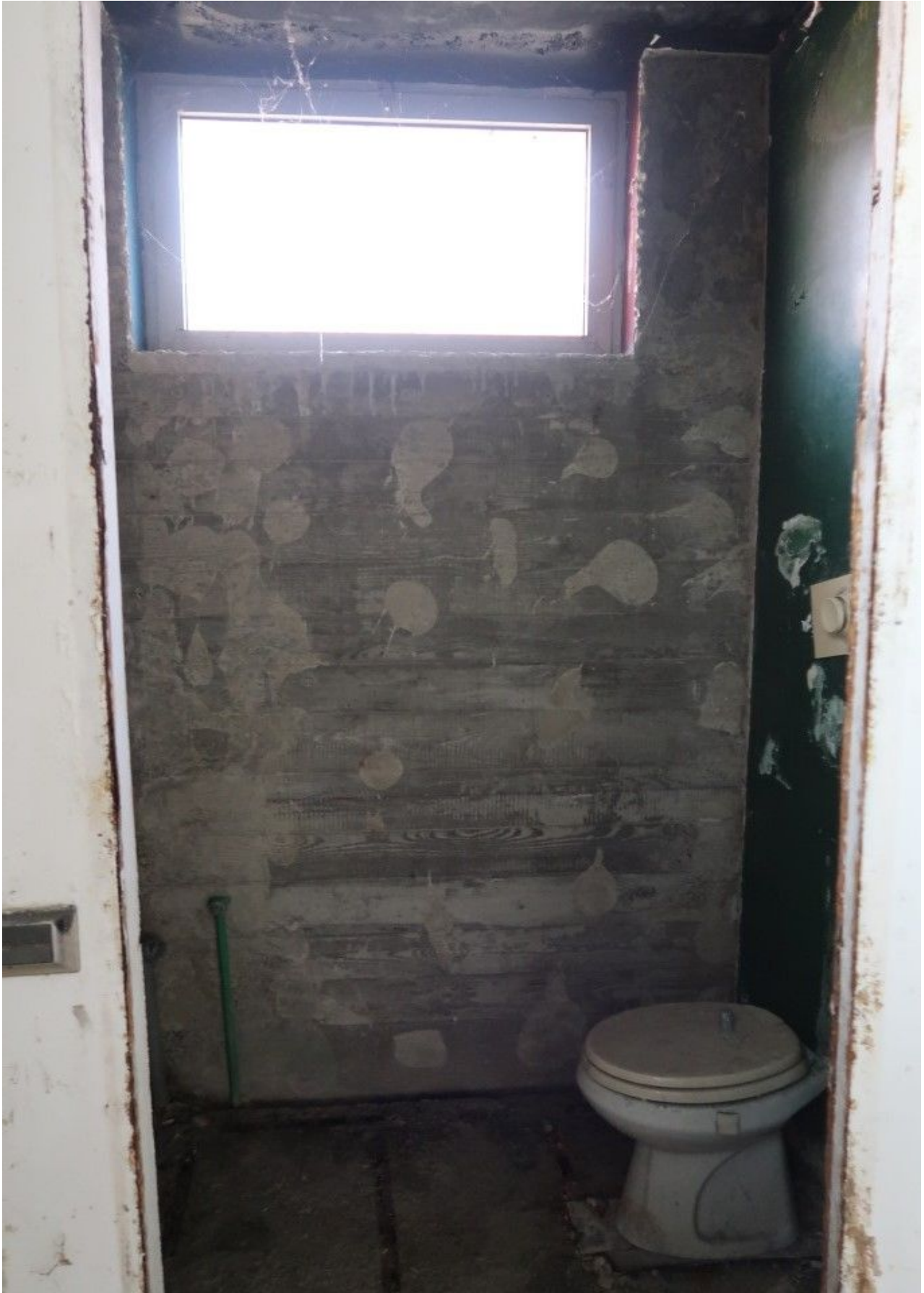
BAGNO PIANO SEMINTERRATO
